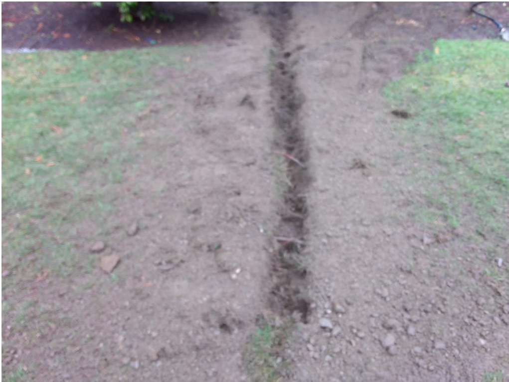
Figure 3. The north trench.
