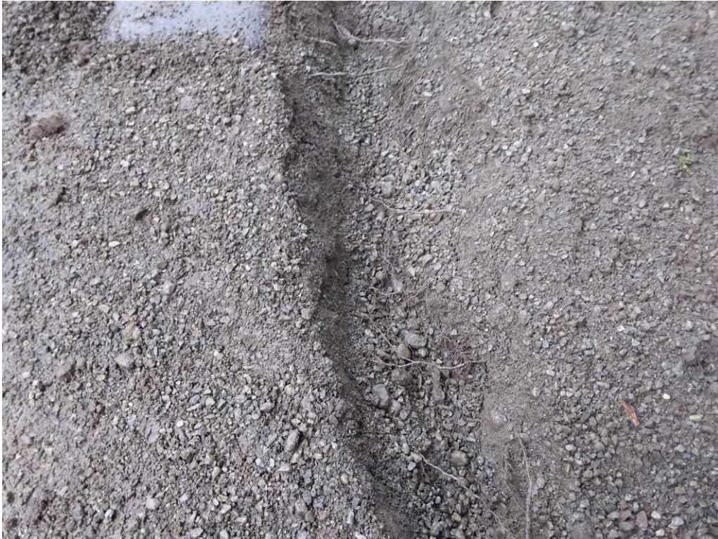
Figure 2. No roots alongside the driveway.
